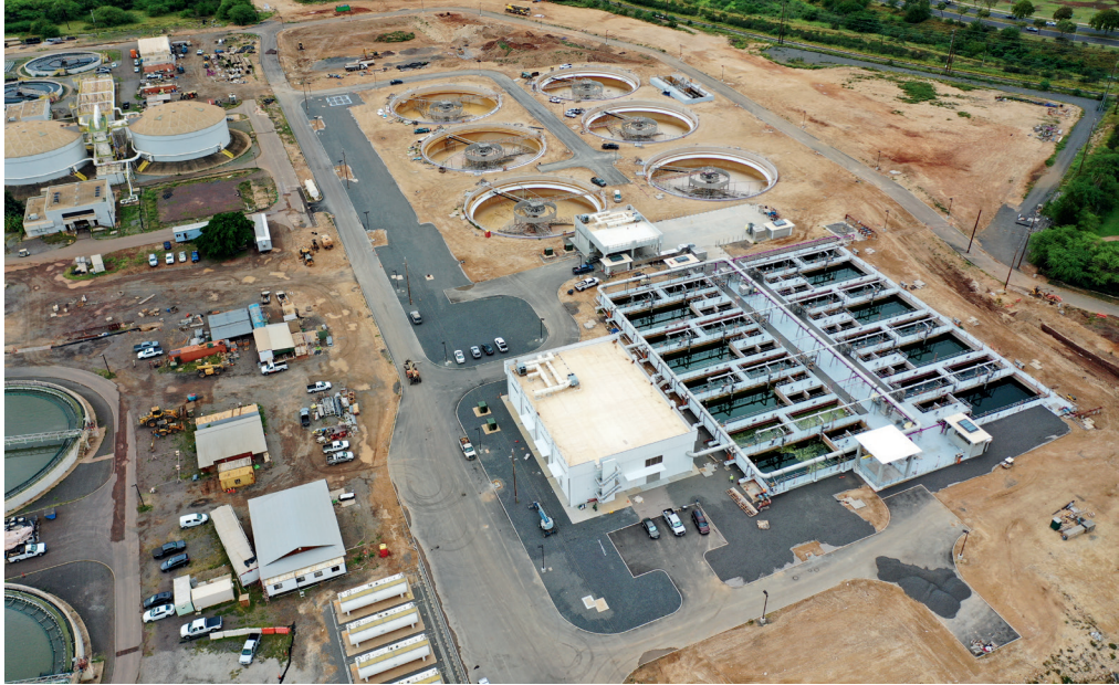
The Honouliuli Wastewater Treatment Plant has achieved full secondary treatment ahead of a federal consent decree deadline. PHOTO COURTESY NAN INC.
